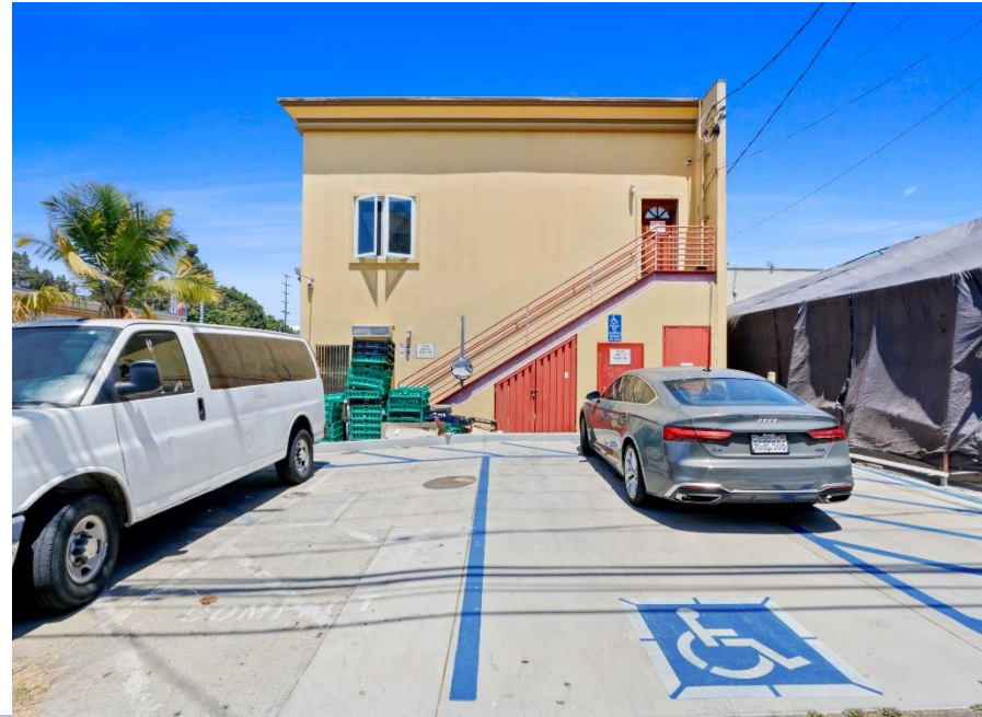
2 nd Floor Office | Storage
